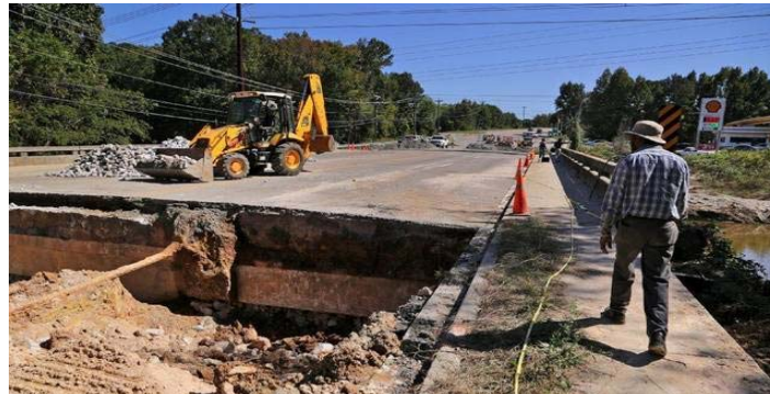
Monticello Road Bridge End Repairs
