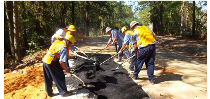
Shoulder and lane repairs
